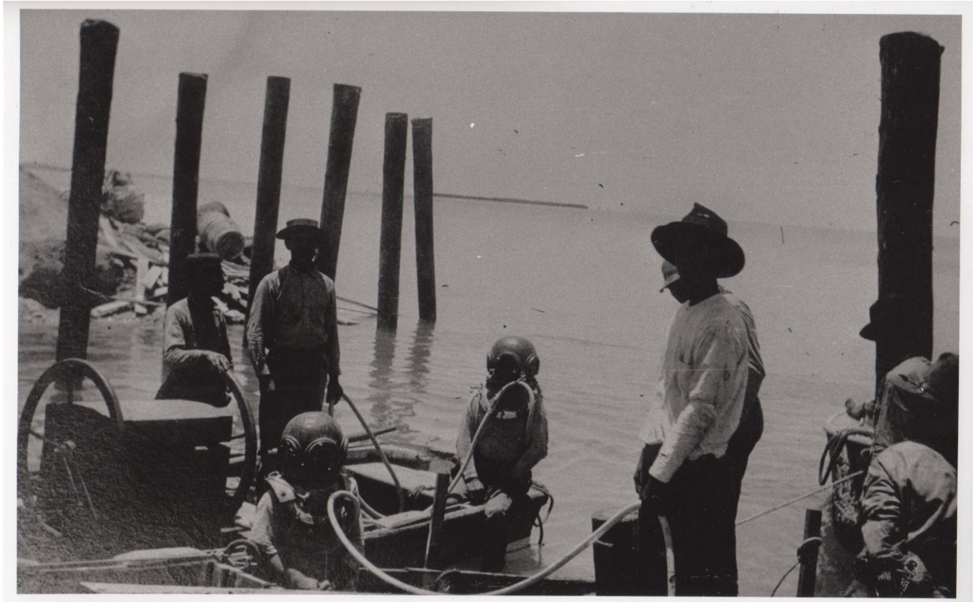
Black and white photograph of hard hat divers working on the bridge piers for the Florida East Coast Railway Company.
