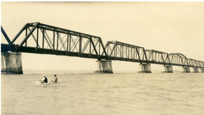
Bahia Honda Bridge, Florida Completed in 1912
