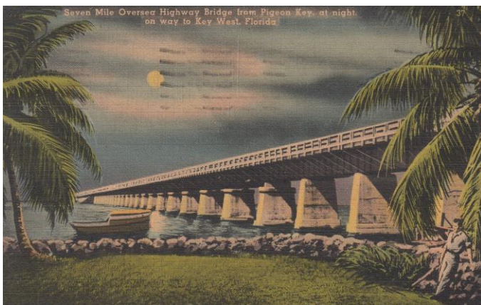
Seven Mile Bridge
