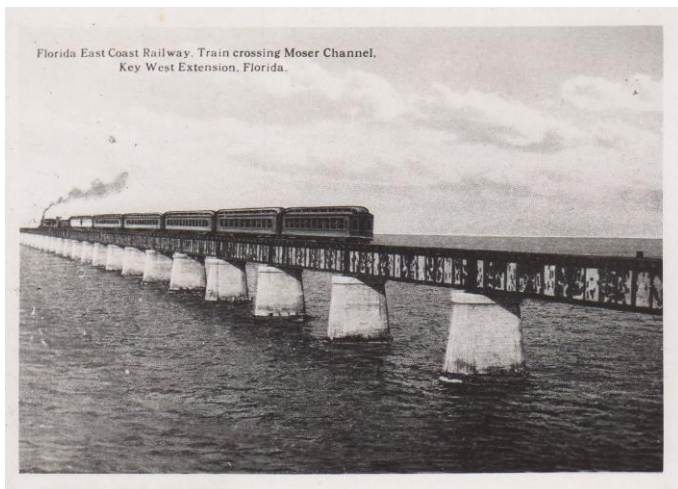
Moser Channel Bridge
