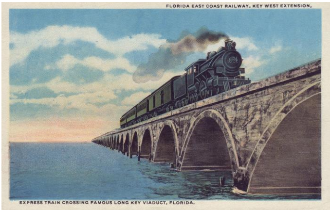
Long Key Viaduct Bridge
